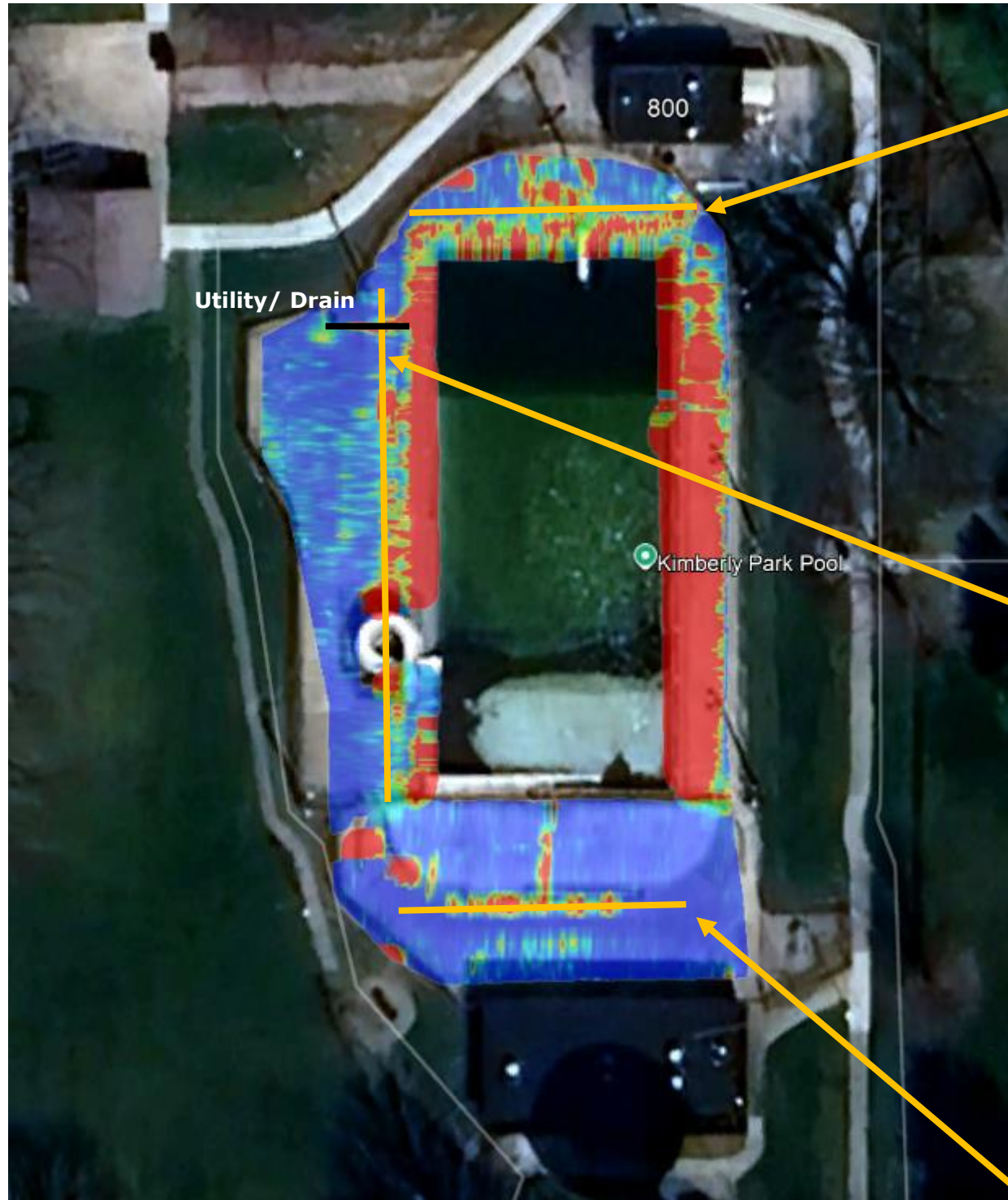
GPR results from outside the pool. Areas of red indicate potential voids, potential water infiltration areas, and potential subsurface moisture or saturation.
