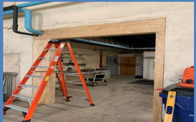
Well Room Roll-up Door Framing
