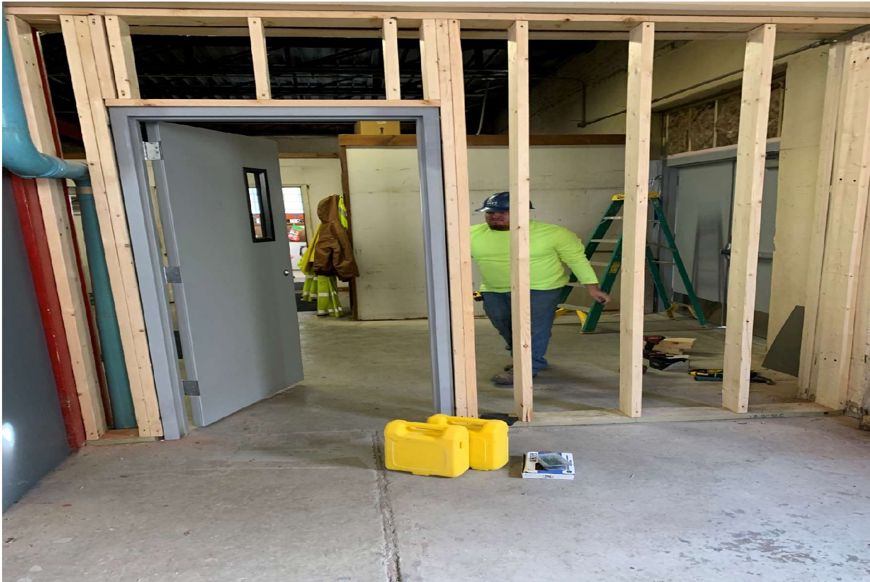
Well 2 Powerhouse Improvements
