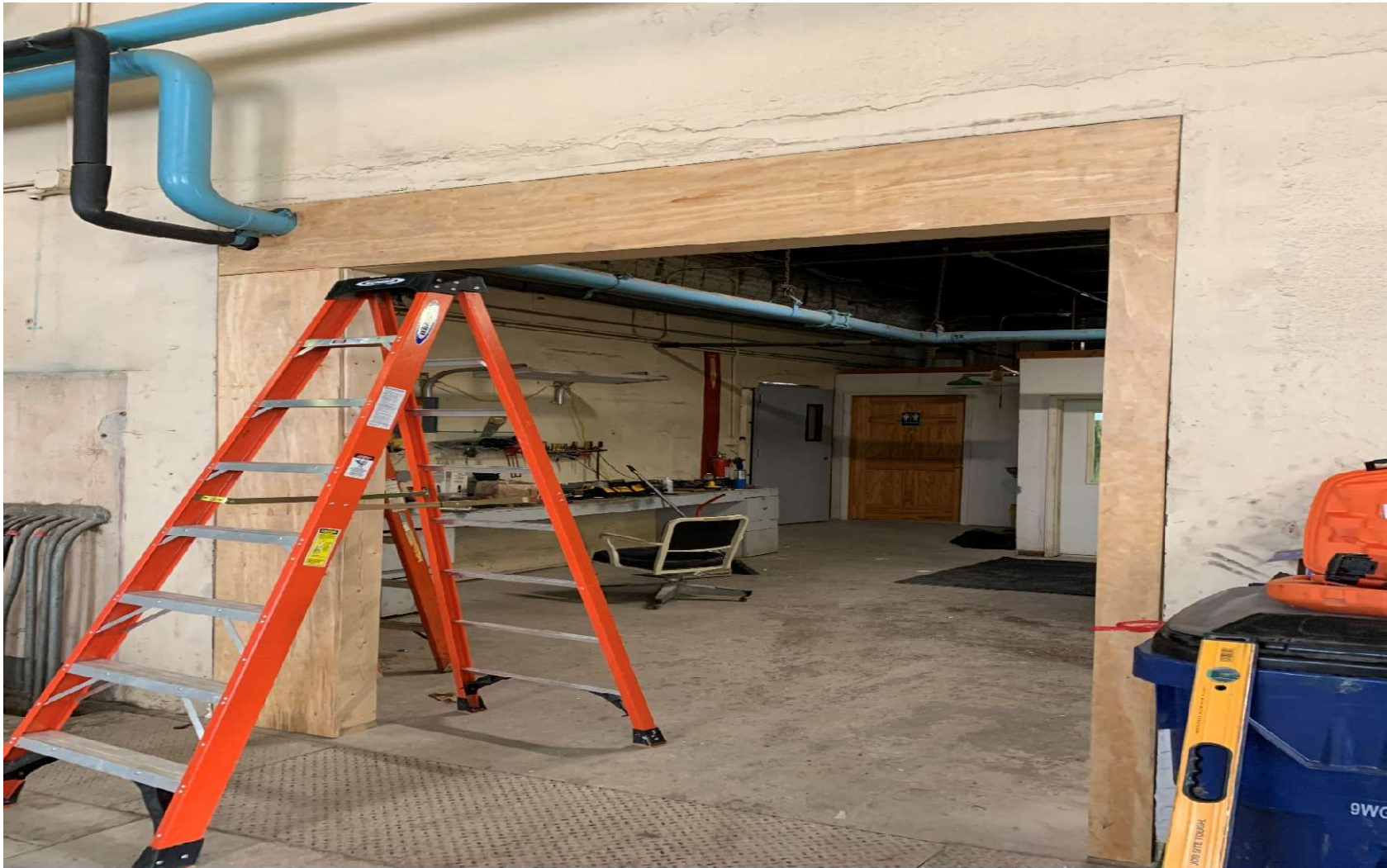
Well Room Roll-up Door Framing
