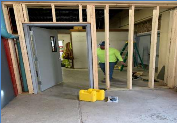
Well 2 Powerhouse Improvements
