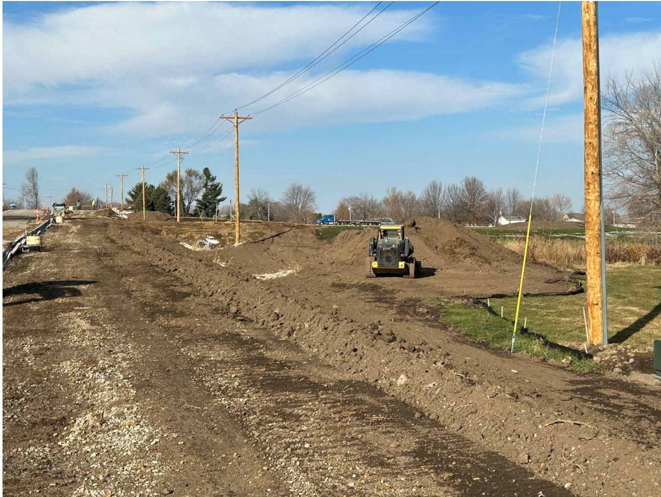
Trail Grading Complete
