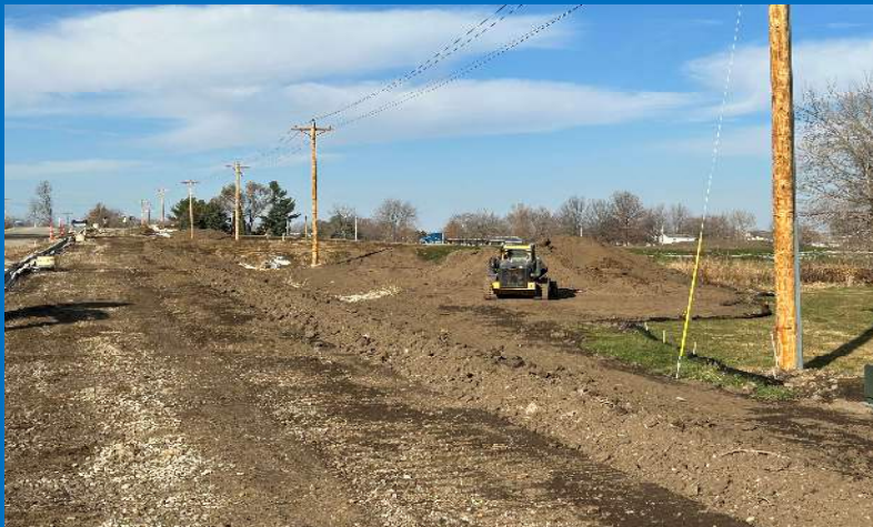
Trail Grading Complete
