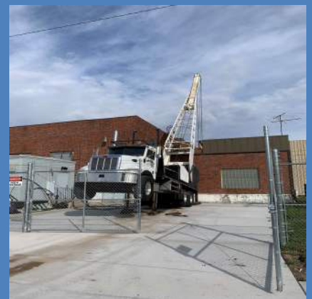
Northway Well Rig in Place
