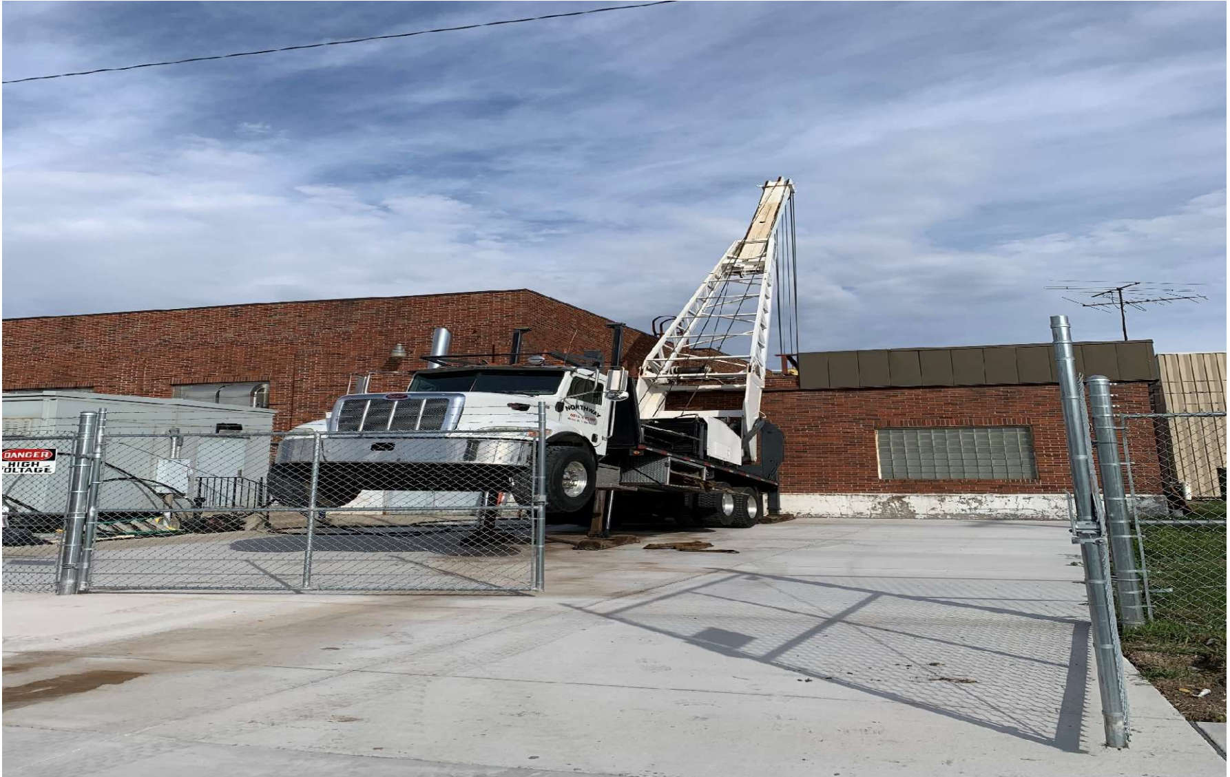
Northway Well Rig in Place
