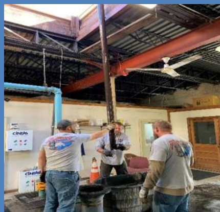
Well No. 2 Cleaning
