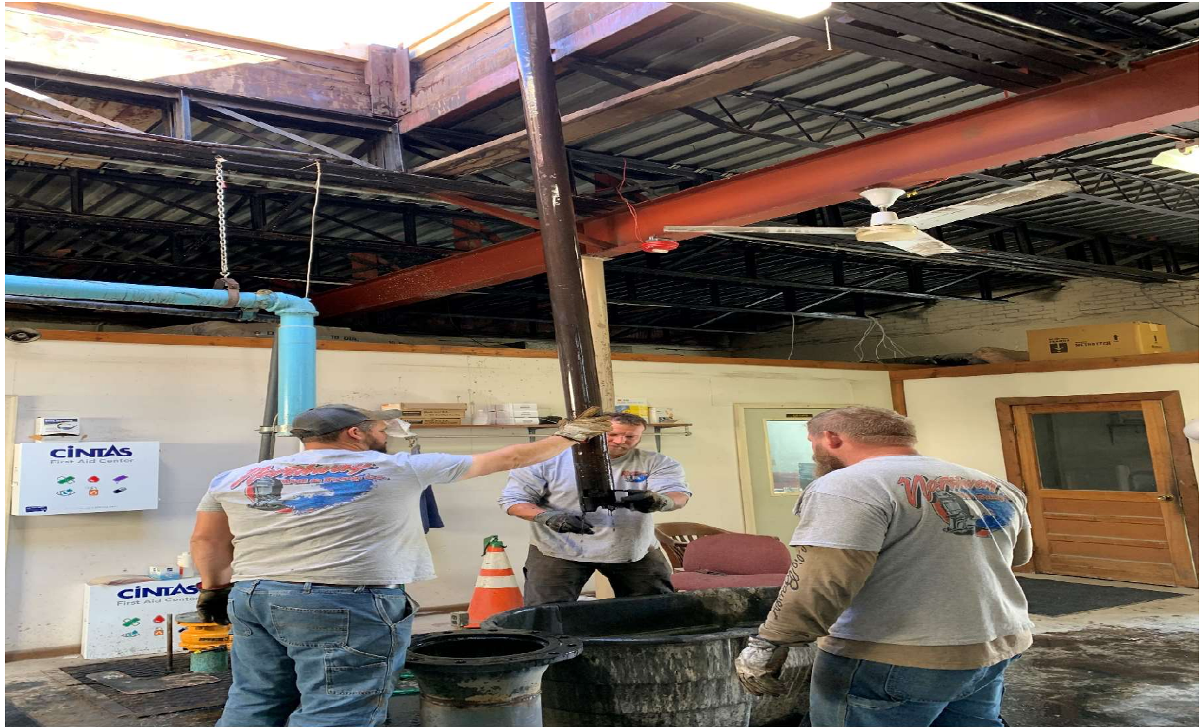
Well No. 2 Cleaning
