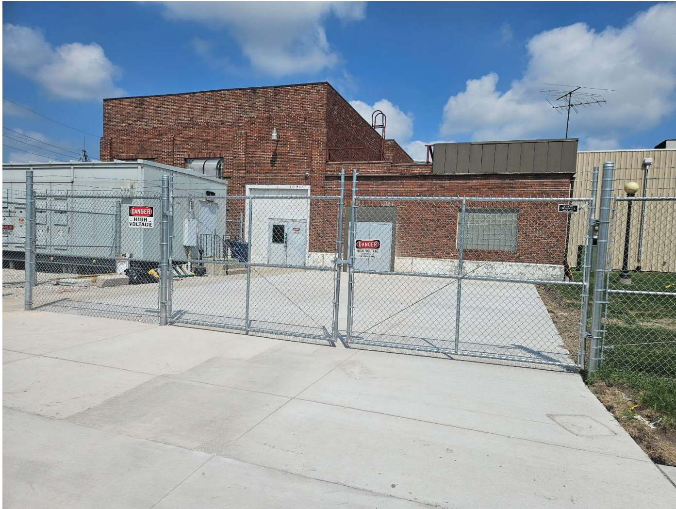
Phase II - New Pumphouse Driveway
