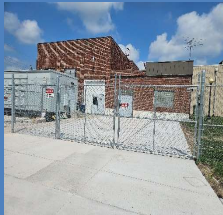
Phase II - New Pumphouse Driveway
