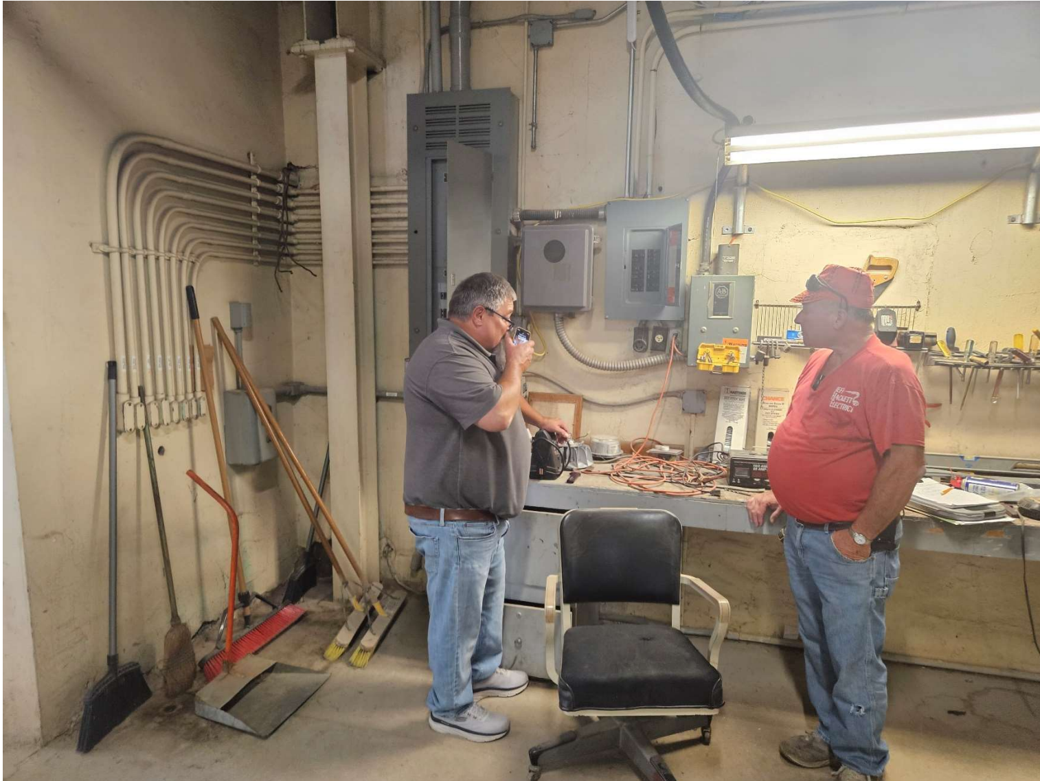
Phase I - Contractors Viewing Electrical Work
