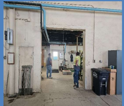
Phase II - Opening for Roll-Up Coil Door
