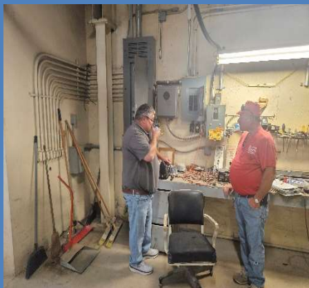
Phase I - Contractors Viewing Electrical Work
