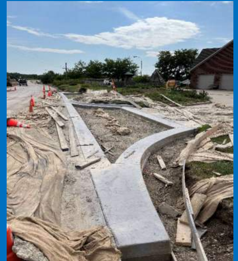
Stamped driveway replacement
