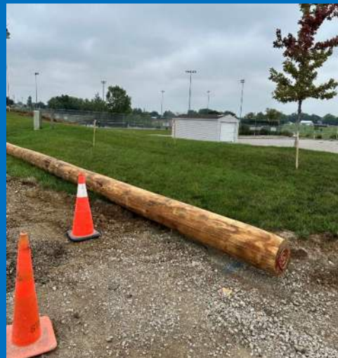
Power Poles Relocation Started
