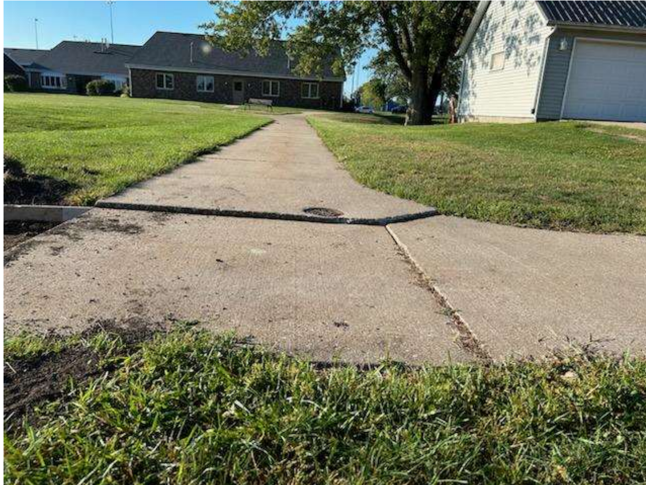
Maxson Avenue Sidewalk Extension
