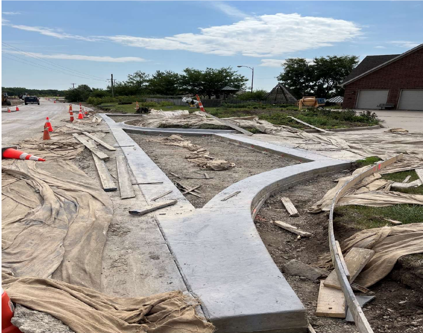
Stamped driveway replacement
