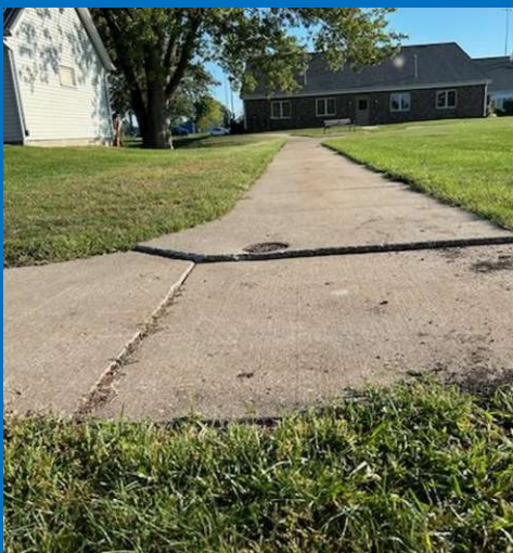
Maxson Avenue Sidewalk Extension
