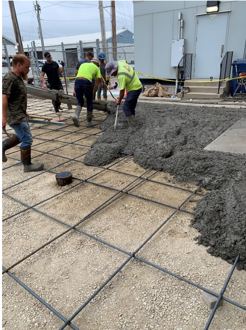
Installation of New Driveway
