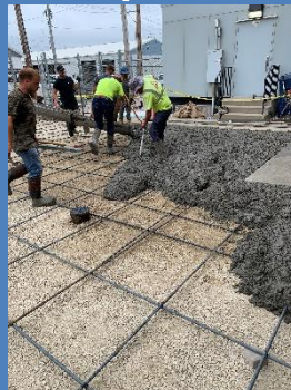
Installation of New Driveway
