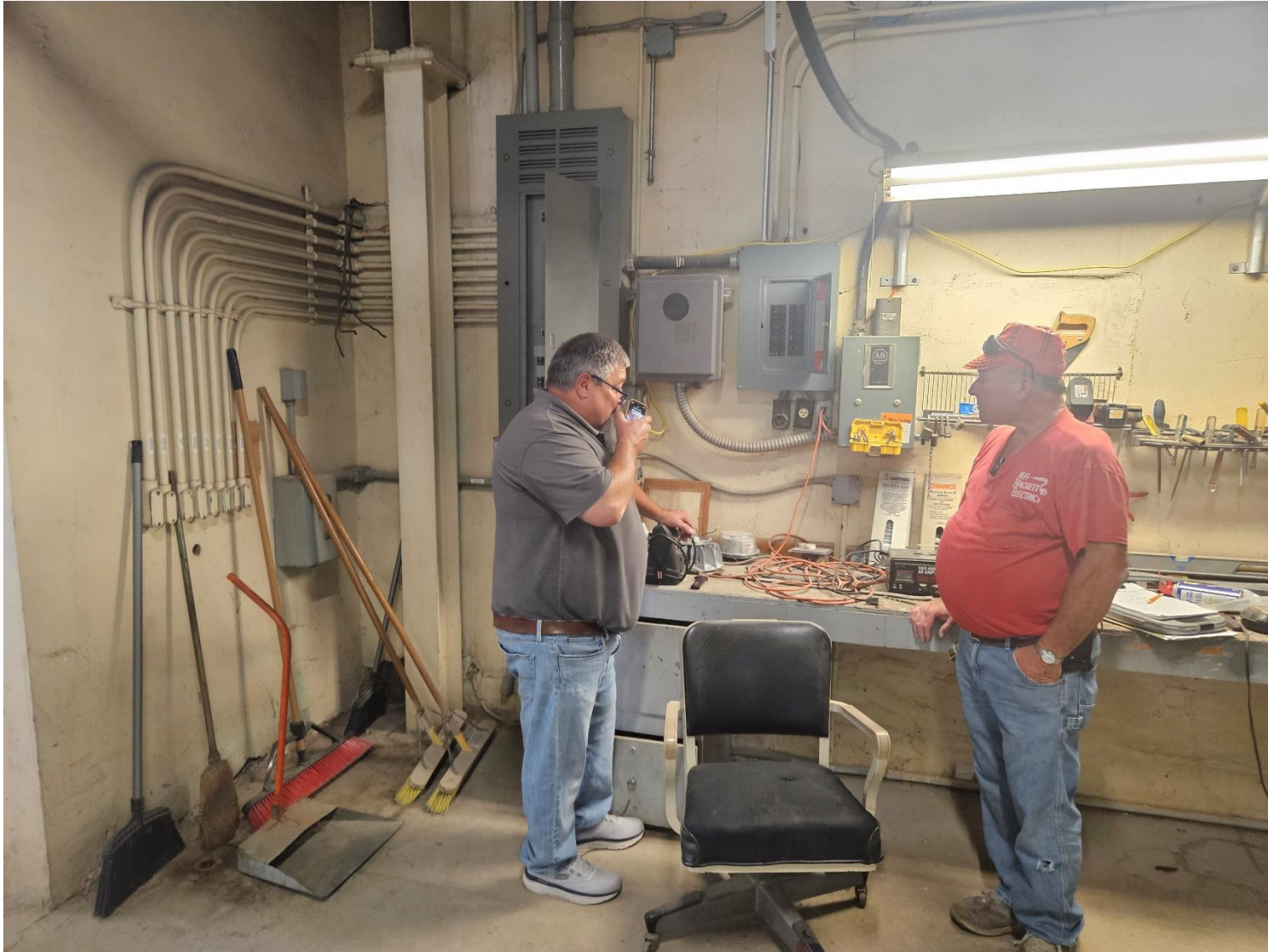
Phase I - Contractors Viewing Electrical Work
