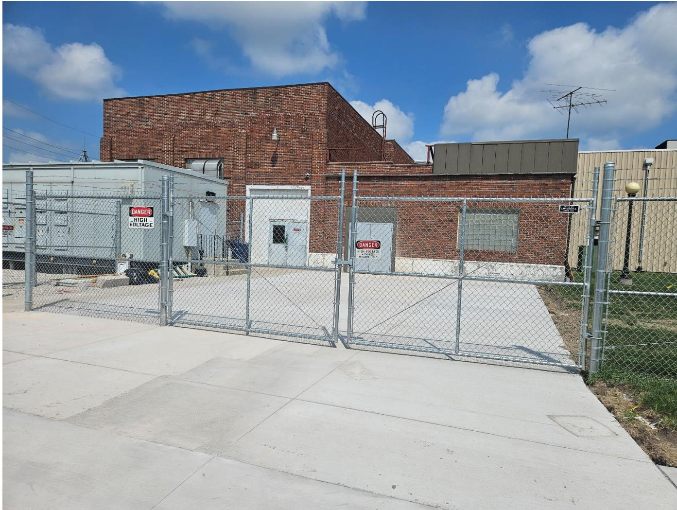
Phase II - New Pumphouse Driveway
