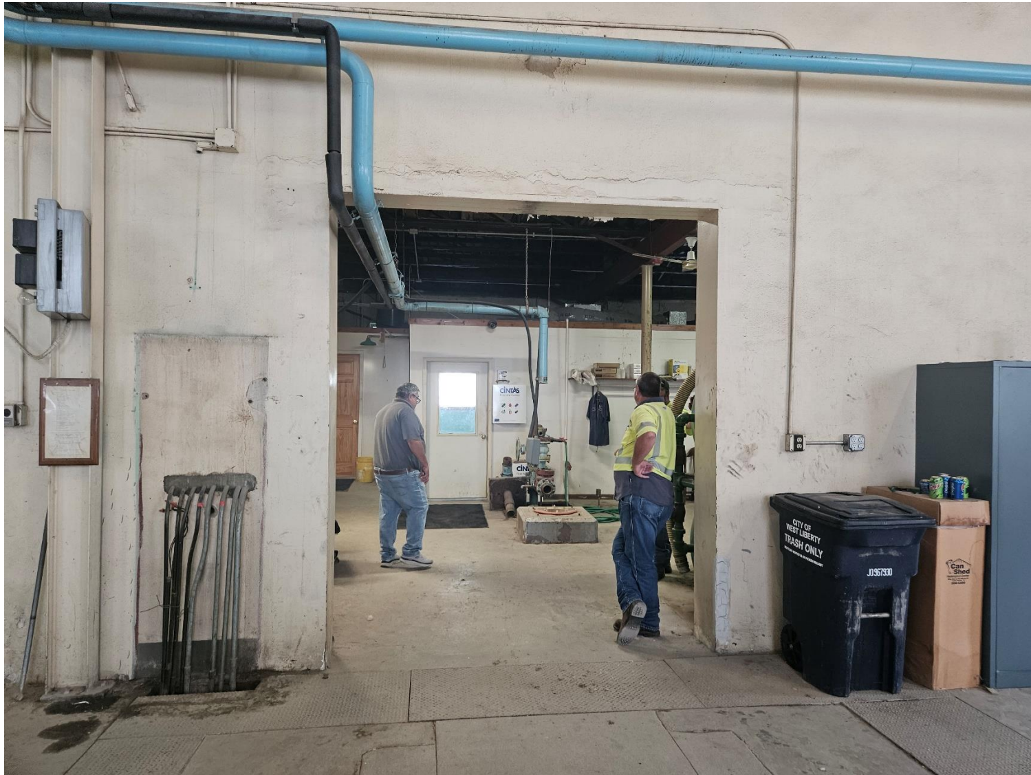
Phase II - Opening for Roll-Up Coil Door
