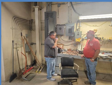
Phase I - Contractors Viewing Electrical Work
