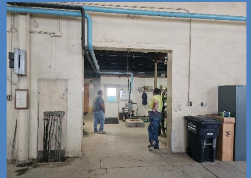
Phase II - Opening for Roll-Up Coil Door
