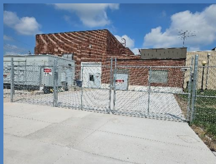
Phase II - New Pumphouse Driveway
