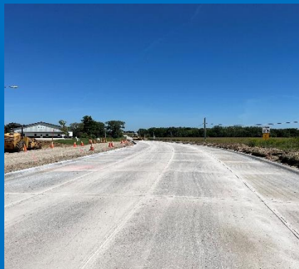
New Road and Trail Grading
