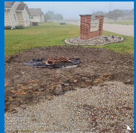
Storm Intake Erosion Control
