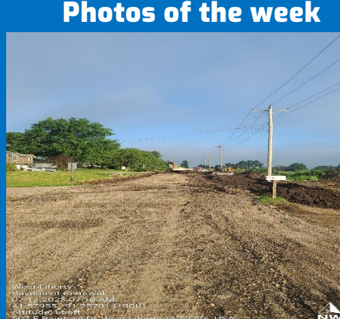
Pavement removal West End Rainbow
