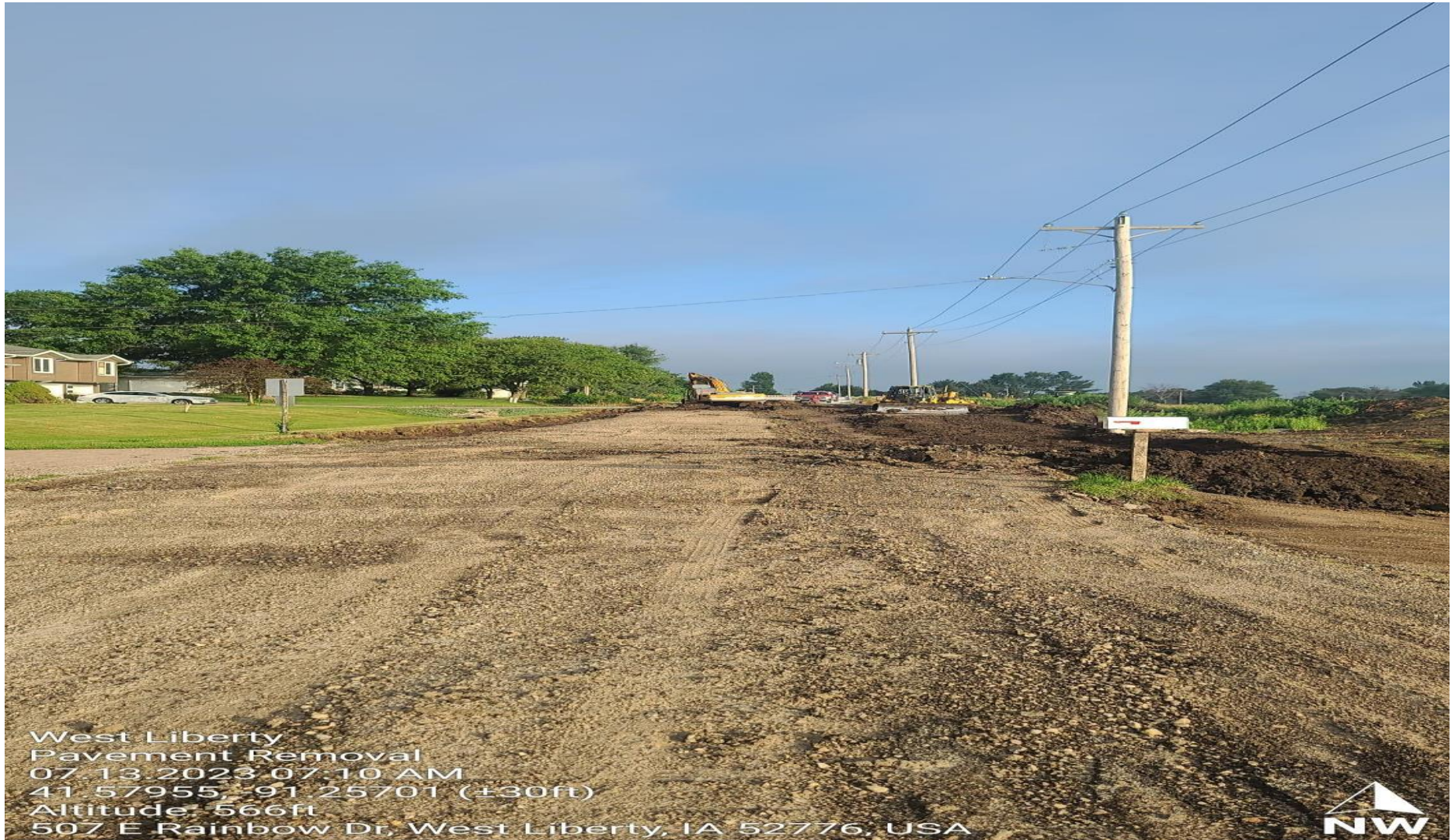
Pavement removal West End Rainbow
