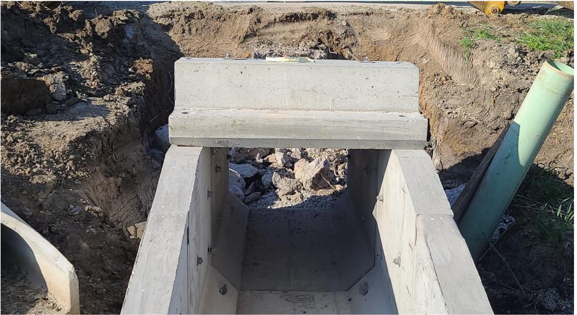
4' X 4' Culvert Installation
