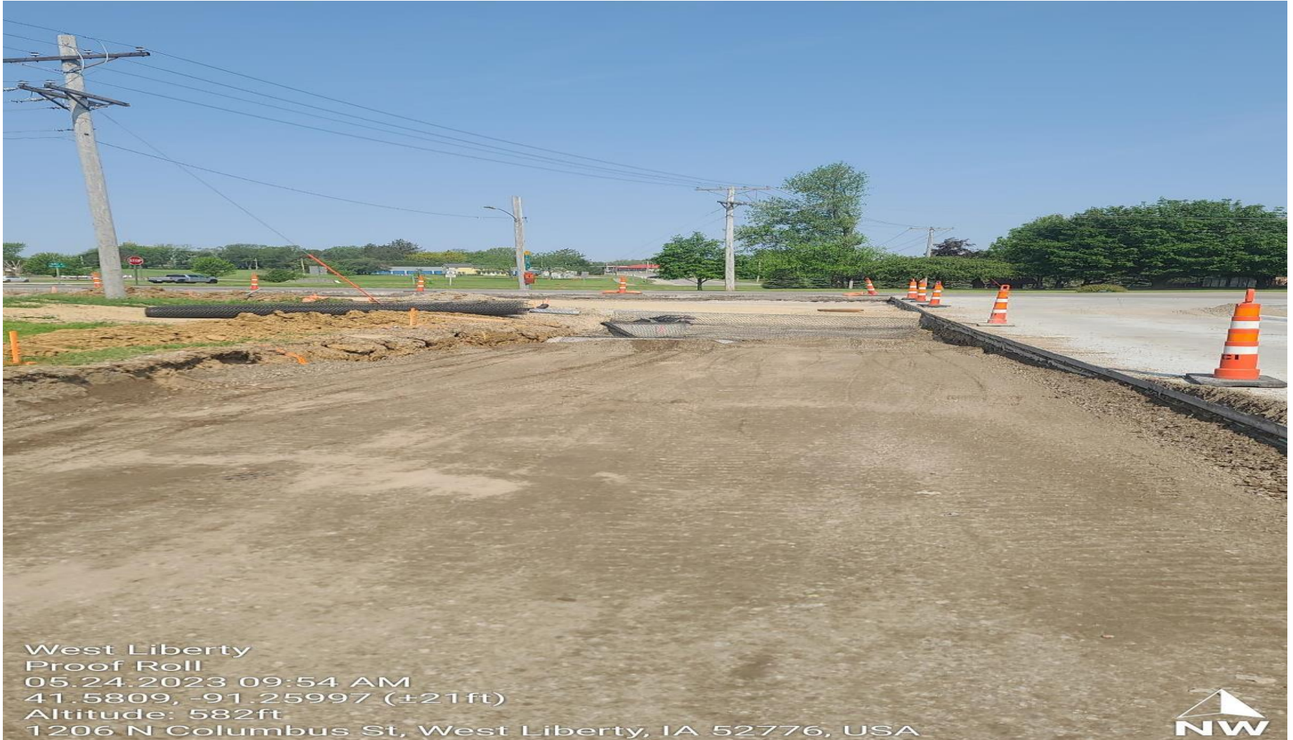
Phase I Subbase after Proof Roll
