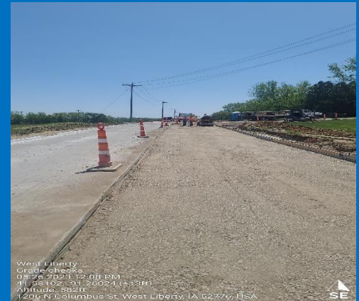
Roadway Concrete Grade Checks
