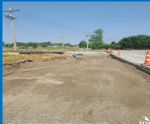
Phase I Subbase after Proof Roll
