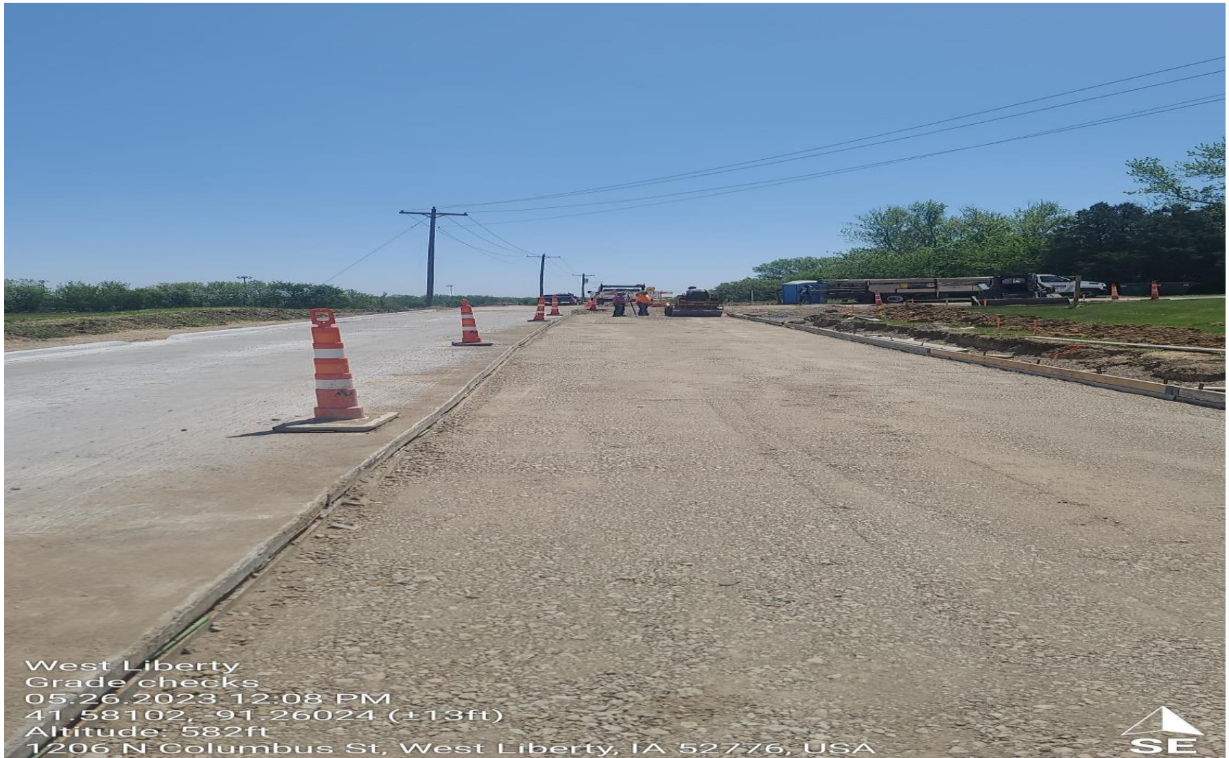
Roadway Concrete Grade Checks
