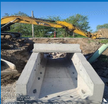
4' x 4' Culvert Installation
