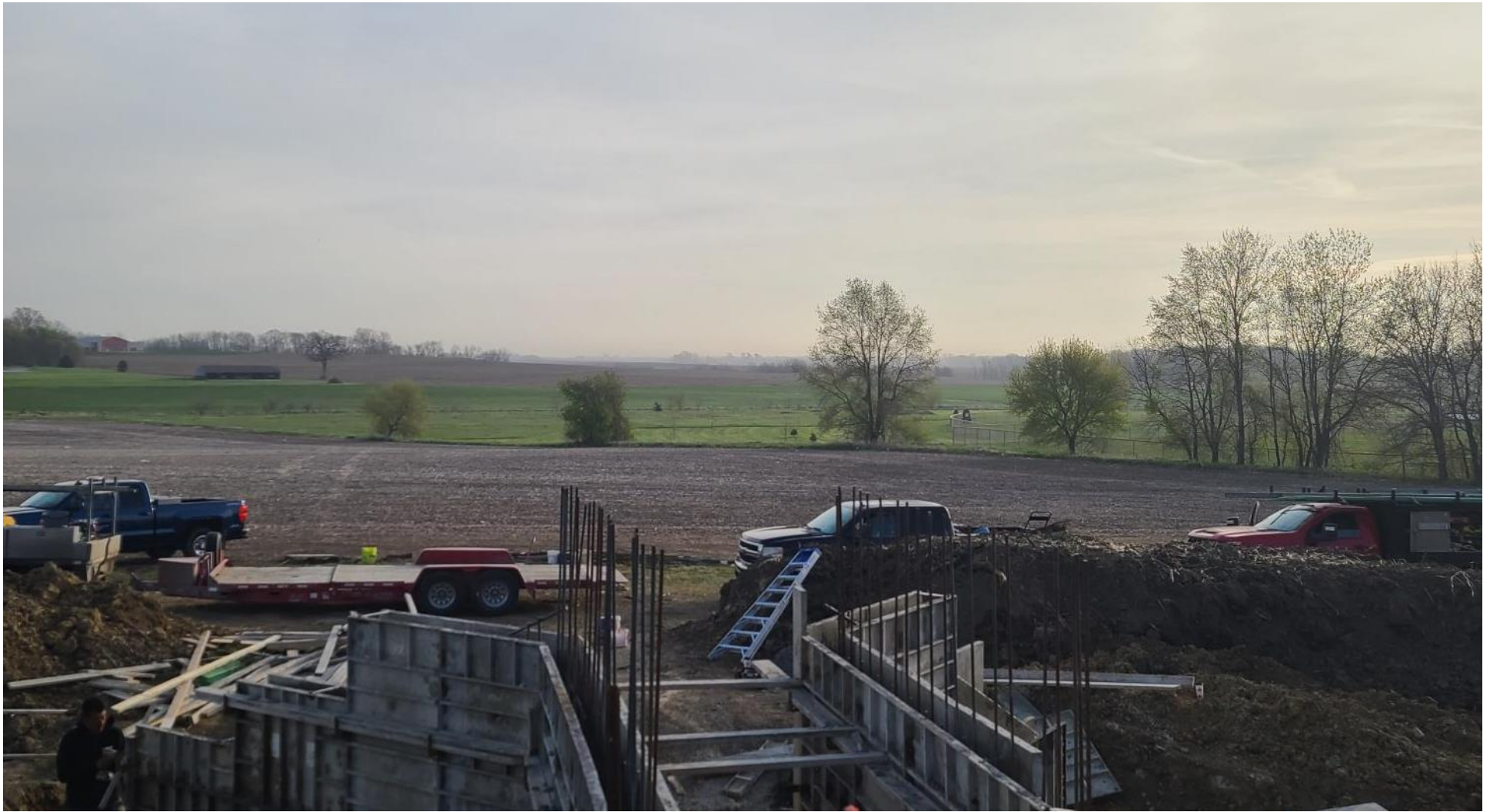
Culvert Ext. Wing Walls Forming for Top
