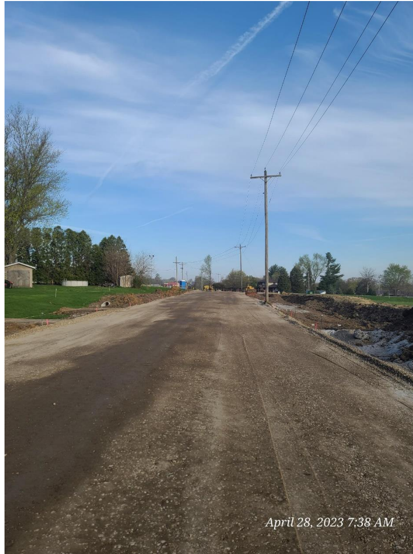
Road Base Rock Installation
