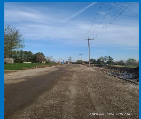
Road Base Rock Installation
