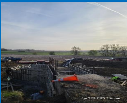
Culvert Ext. Wing Walls Forming for Top
