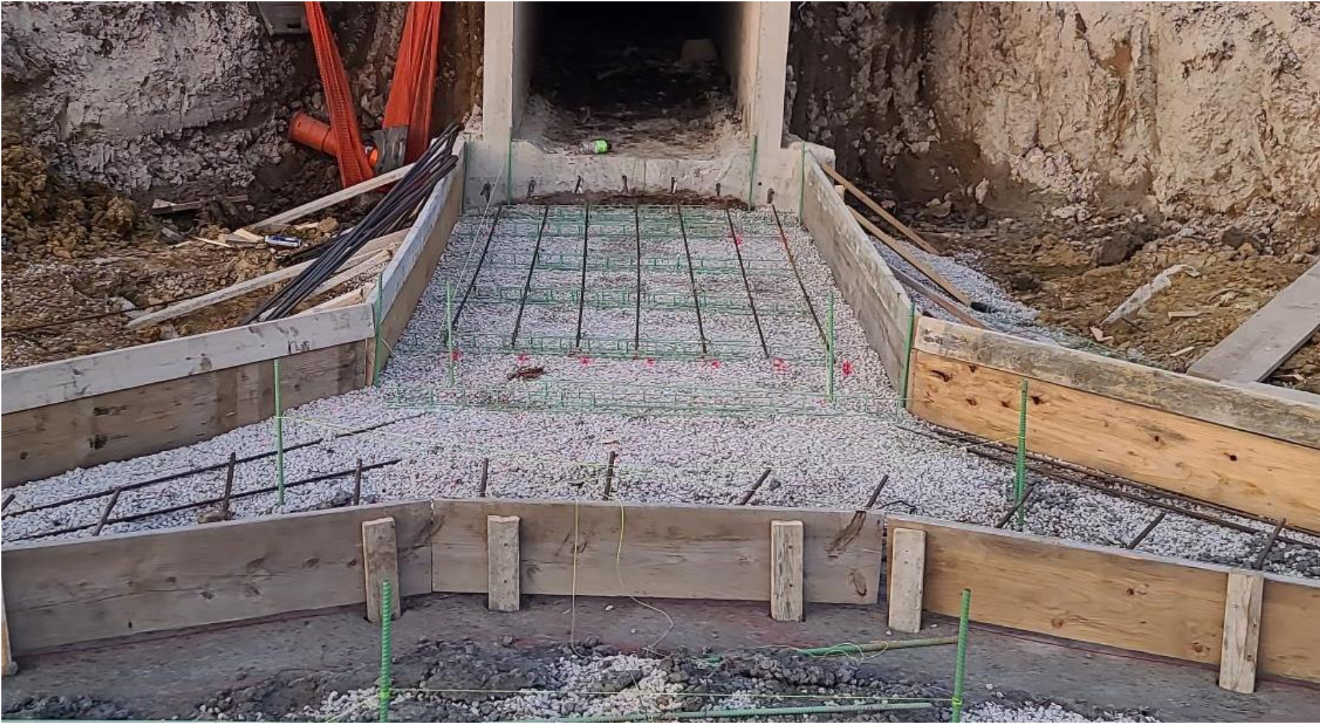
Box Culvert Extension
