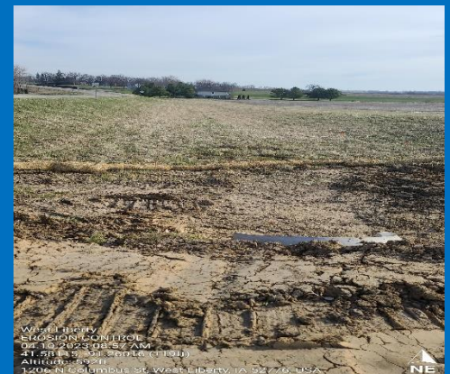
Erosion Control Installed
