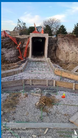
Box Culvert Construction
