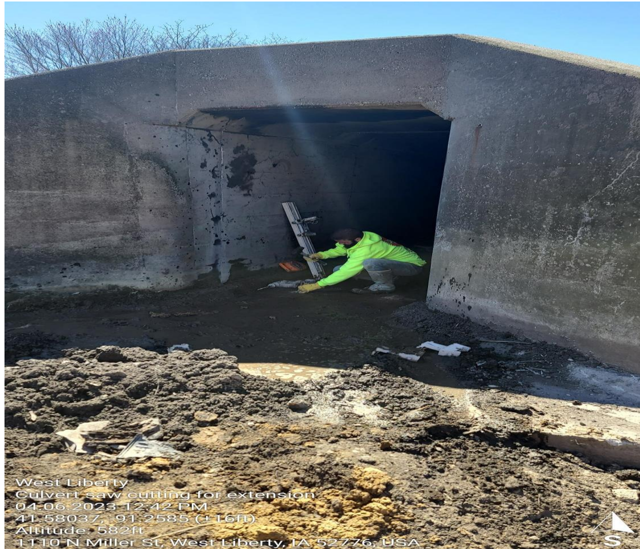
Box Culvert Extension
